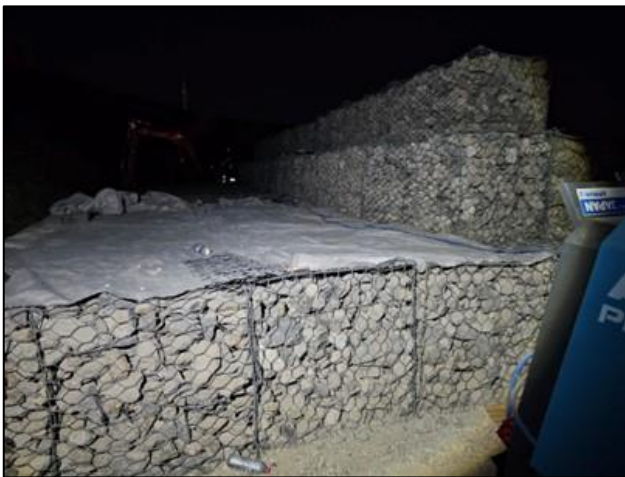
Plate 3. Gabion Baskets in the north-west of the GGF Offset Area (Ecology and Heritage Partners Pty Ltd 21/02/2024).
