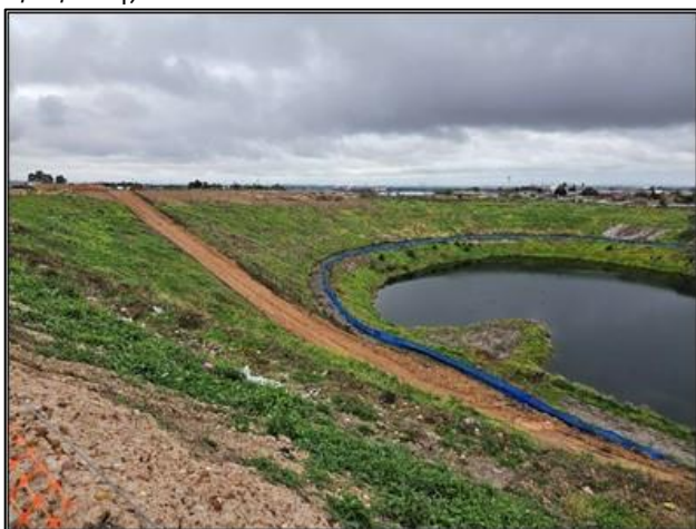
Plate 5. Access track into Offset Area with adjacent frog fencing (Ecology and Heritage Partners Pty Ltd 30/08/2023).
