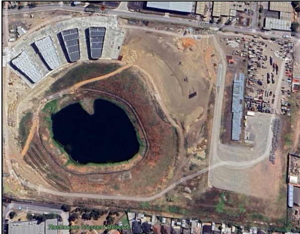
Plate 1. The study area with construction occurring in stages A1-A4 (Google Earth 2024).
