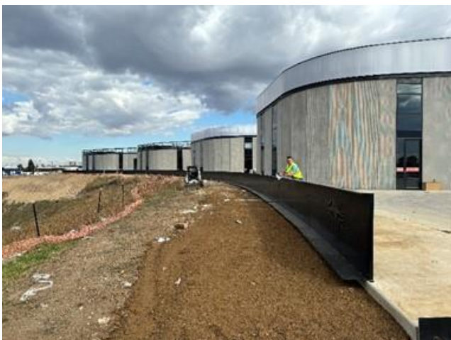
Plate 15. Permanent frog fence installed south of Stage 1. (Forte Group 19/03/2024)
